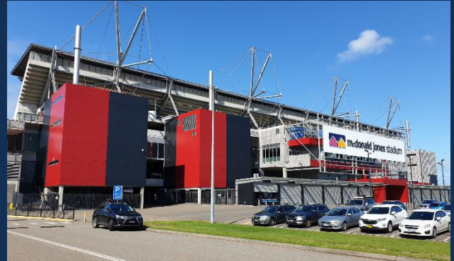
Above: BOSS FacadeGard™ used at MacDonald Jones Stadium Newcastle.
