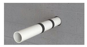
4. Place additional layer(s) of wrap around the pipe or insulation if required, depending on your pipe or insulation size, and secure again with adhesive tape.
