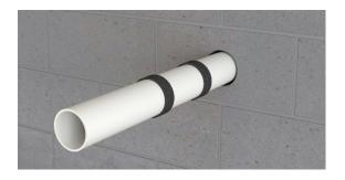
5. Push the UniWrap® into the annular gap between the wall opening and the pipe. Adjust the position of the wrap so that the edge is in line with the wall or floor surface on both sides. Seal over the top of the annular gap with FireMastic-300 in accordance with the approved system application.
